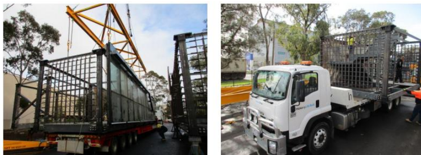
Figure 5. Module Hoisting and Transportation
