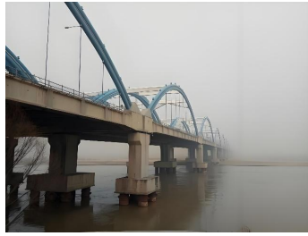
Figure 3. Liujiang Yellow River Highway Bridge
